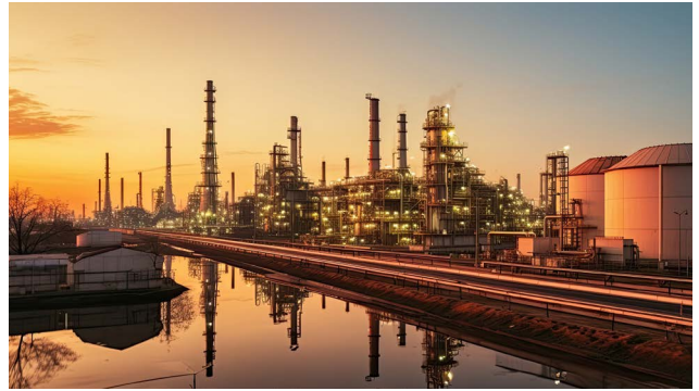
Process and cooling water in chemical plants and refineries.
