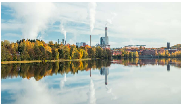
Process and cooling water in the paper industry and other industries.
