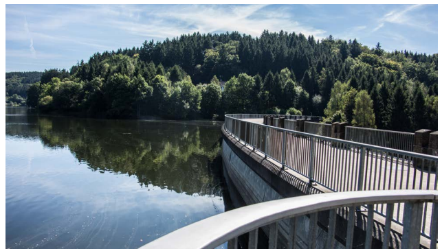
Raw water for drinking water supply.
