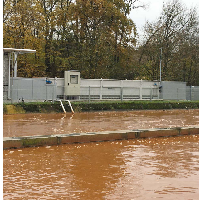
HUBER Dissolved Air Flotation systems for sludge separation and effluent treatment – the solution for upgrading overloaded wastewater treatment plants.
