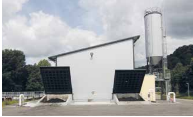
Sludge bunker and dry material silo.
