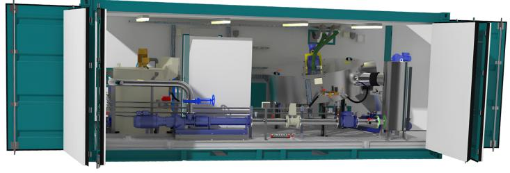
The containerised HUBER S-DISC sludge thickening plant was a design concept that HUBER GB developed during the COVID lockdown, achieving the first sale in 2022. It's not a trial unit but a fully WIMES compliant maintainable package plant that includes the S-DISC thickener, feed and discharge pumps, a bunded poly make up & dosing unit, heating, lighting and ventilation and a WIMES 3.04 control panel built in-house to each water company specification.
