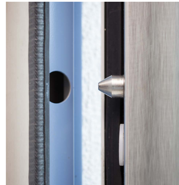
Detailed view of anchor bolts.
